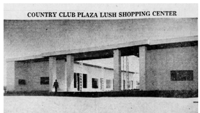
Country Club Plaza Lush Shopping Center, Tucson (Foto: Arizona Daily Star, 9.10.1946)
